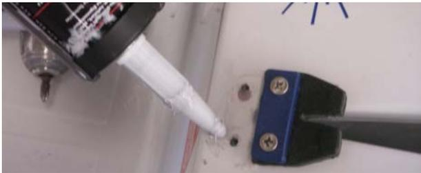
2 Apply a sealant to the screw holes.
